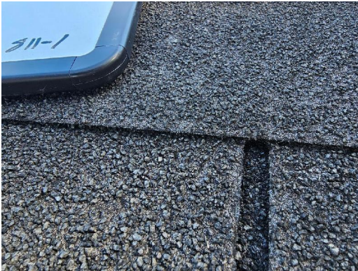
811-1 Asphalt Shingle/Tar Typical Exterior Roof
