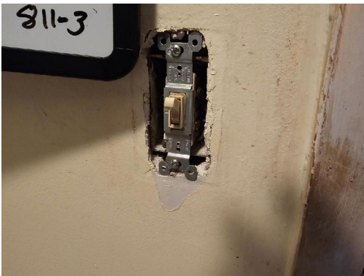
811-3 Drywall/Joint Compound Typical Interior Walls/Ceilings
